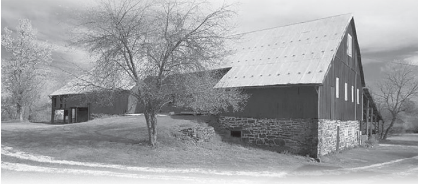
The historic Crawford Barn, not far from the Gettysburg Battlefield, has been carefully restored and maintained over the last several decades by Gabor and Elizabeth Boritt. In 2018, it received a HGAC Barn Preservation Grant to help rebuild one of the barn's walls.
